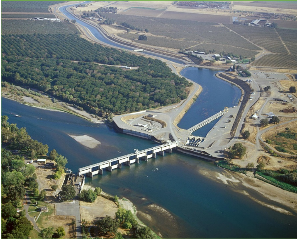
Figure 27: The Junction of the Red Bluff Diversion Dam and the Tehama-Colusa Canal along the Sacramento River in Red Bluff. Due to fish passage improvement, the Dam gates are now permanently open. The Tehama-Colusa Canal Authority operates and maintains the 140 mile Tehama-Colusa and Corning canals irrigation water supply system. Source: Bureau of Reclamation.
