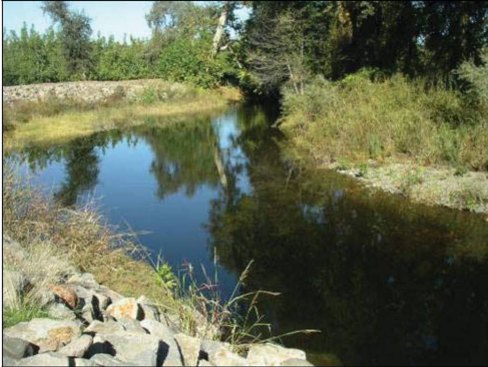
Figure C-39. Levees and riprap along channel banks in Reach 1 of Craig Creek.
