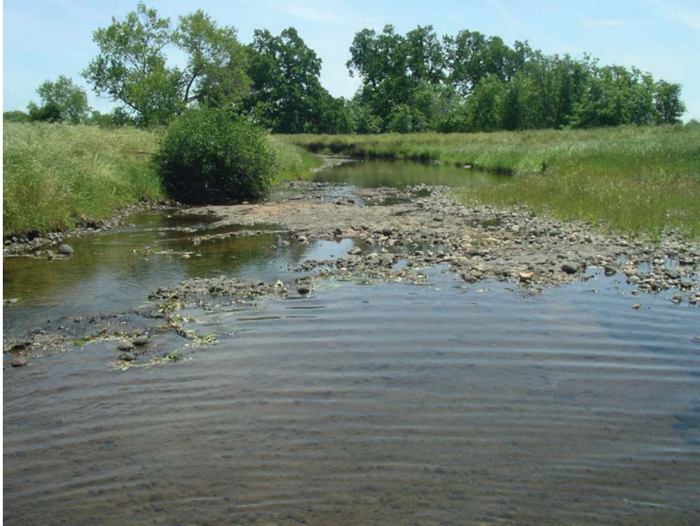
Figure C-17. Potential barrier A1.1 (spring 2010). A wide, shallow bedrock channel segment forming a potential barrier in Reach 2 of Antelope Creek.
