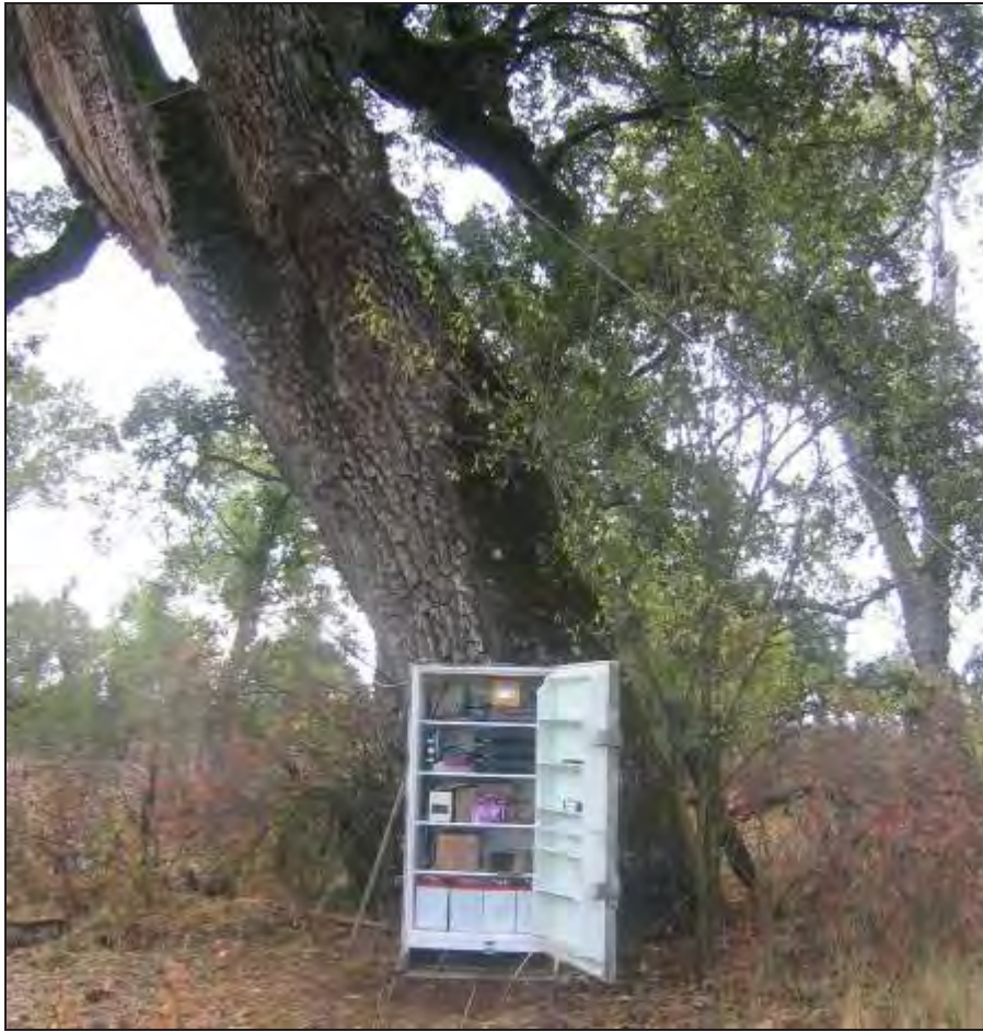
Figure 7. The modified refrigerator contained the DVR's, power controls, equipment and storage boxes, monitor and batteries. The cable above the lock box is the anchoring cable to the two main cables suspending the camera over the creek.
