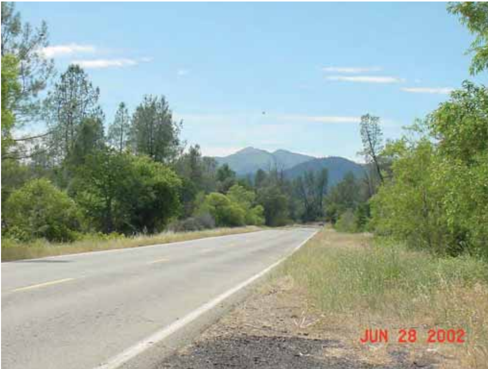
Clear Creek Rd, btwn Gas Point & CCW NE boundary. (PROPOSED PROJECT AREA F)
