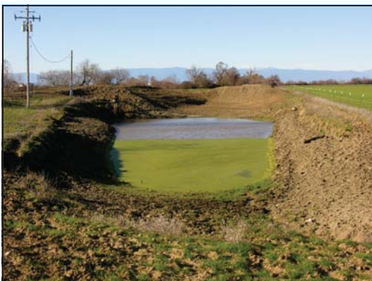
Tailwater pond after excavation
