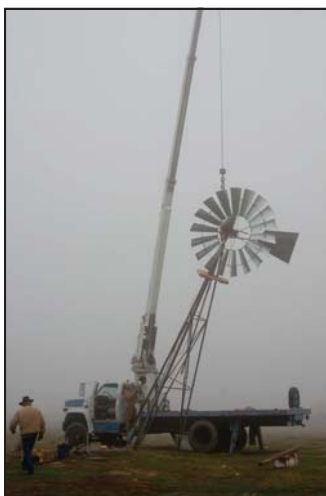
Installing windmill.
