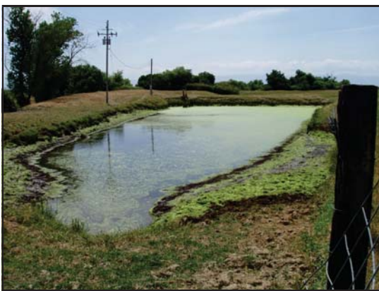
A tailwater pond before excavation to increase its capacity.
